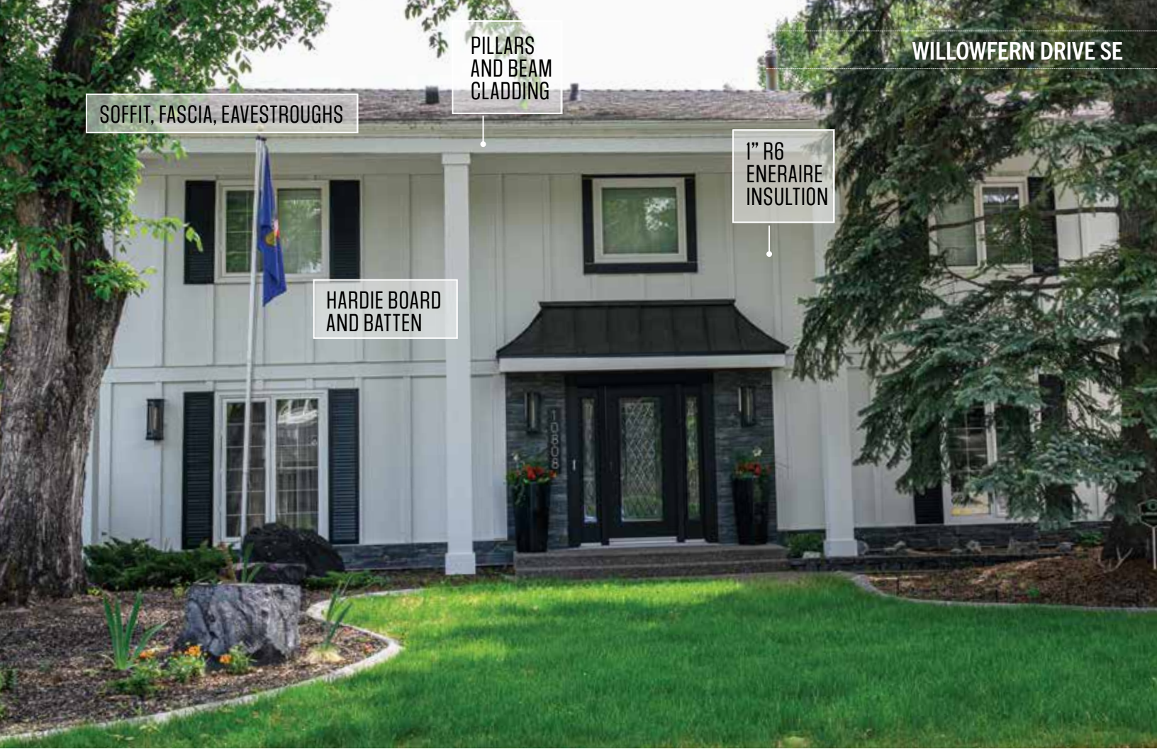
ENTRY DOOR OVERHANG ADDITION WITH STANDING SEAM METAL ROOF WITH CEDAR SOFFIT AND POT LIGHTS
